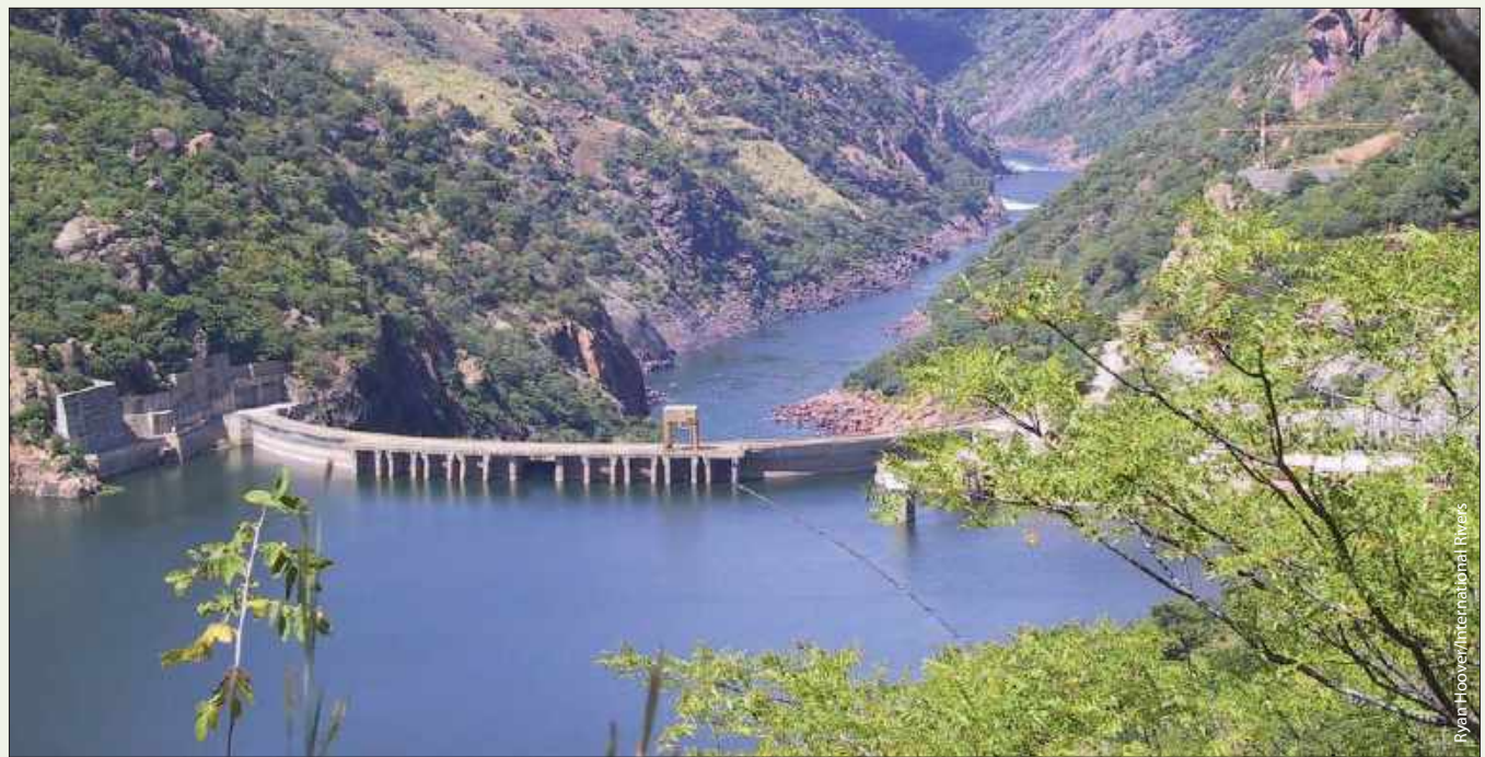
Cahora Bassa Dam in western Mozambique
