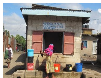
Water kiosk obtaining water from nearby borehole
