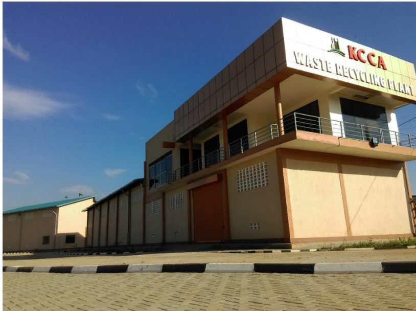
model waste recycling plant for KCCA- process 40,000 tonnes of plastic and 1,000 tons of market waste/mo- LVEMP II
