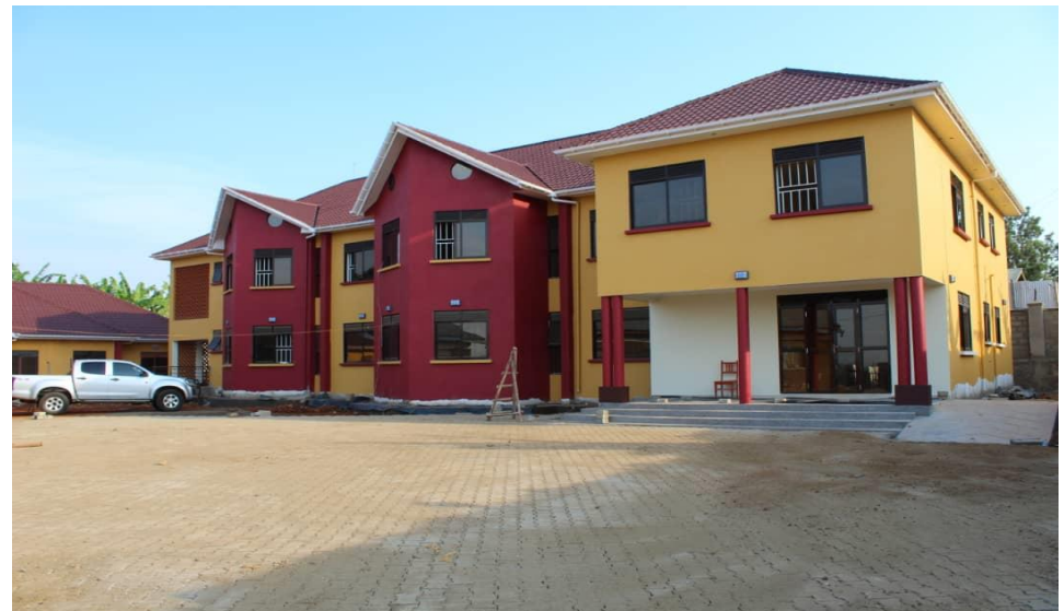
Regional Water Quality Laboratory Block for Albert Water Management Zone - LEAF
