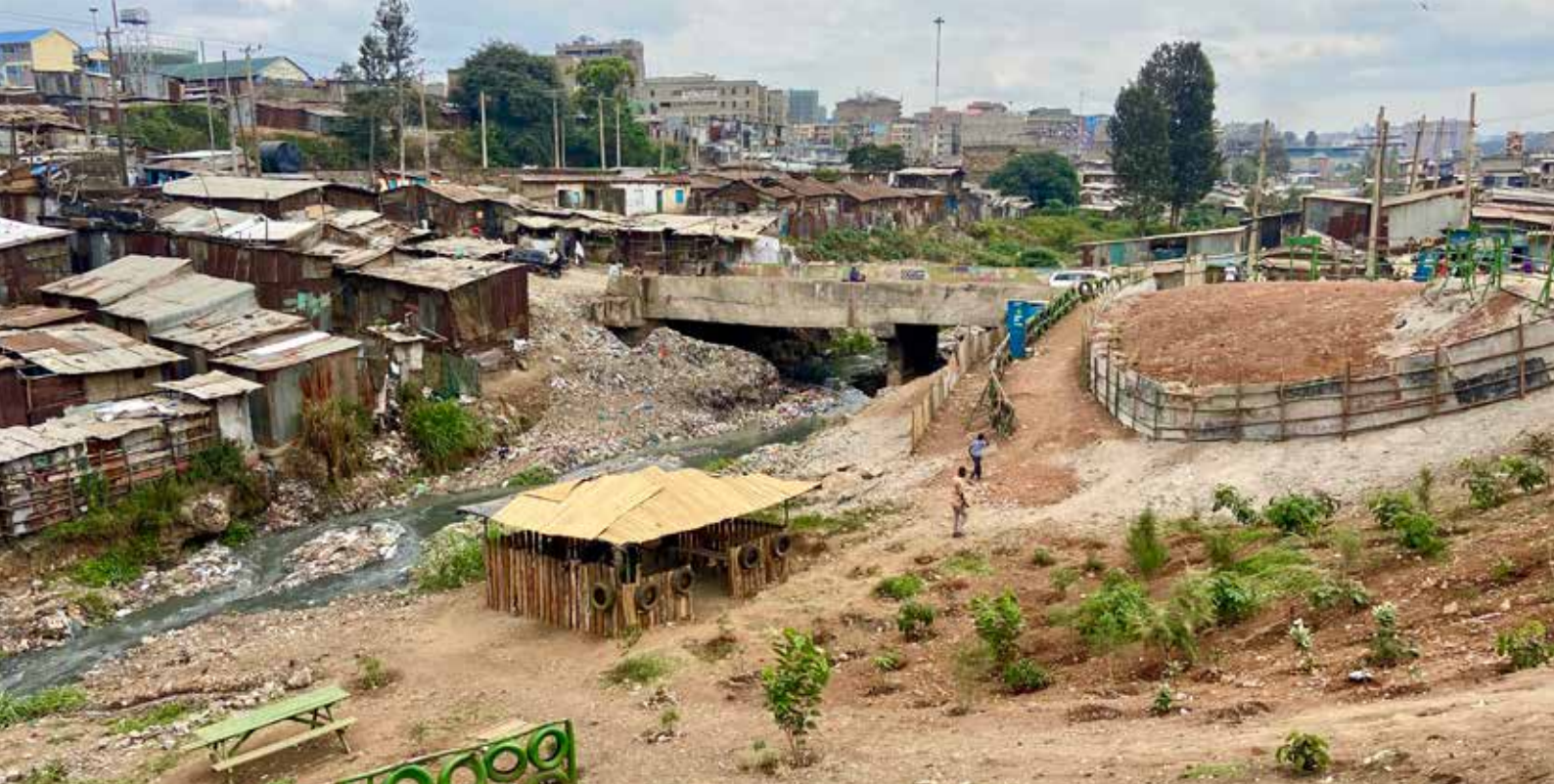
A new community park in Mathare has transformed a former dump site into an urban forest and gathering space alongside the Mathare River, created by the Itals and Masca coalition of youth groups, with support from many others.
